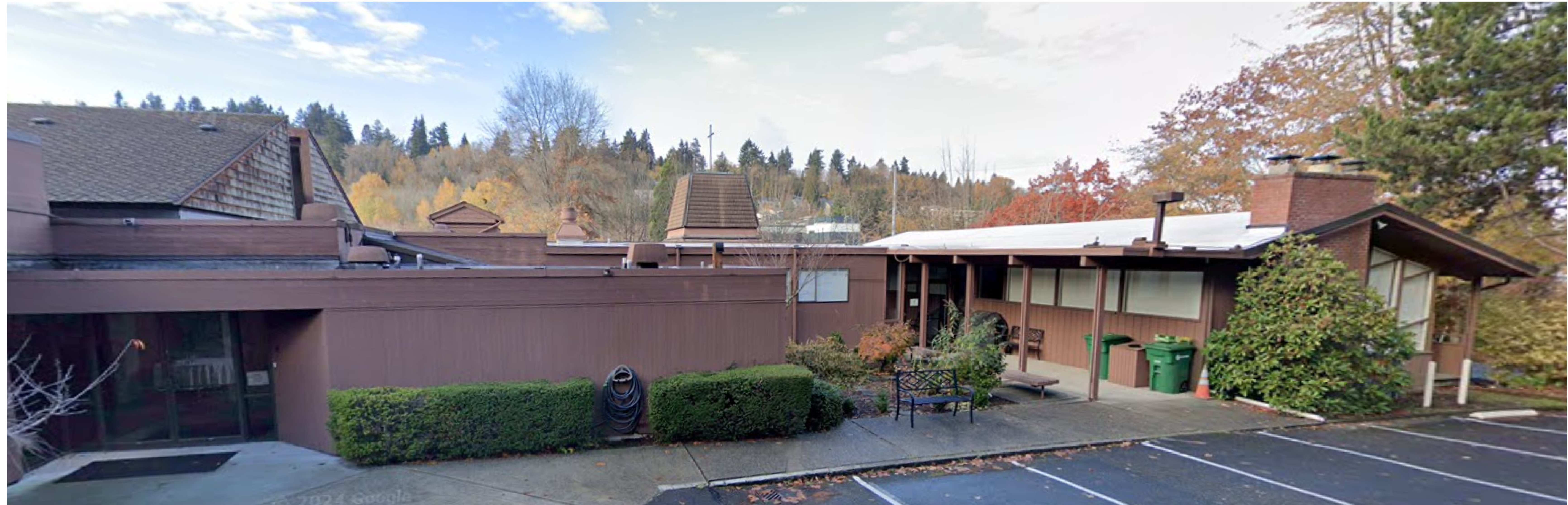
EASTERN PARKING LOT VIEW - FACING FIRESIDE ROOM AND ENTRANCE TO SECOND FLOOR CLASSROOMS
