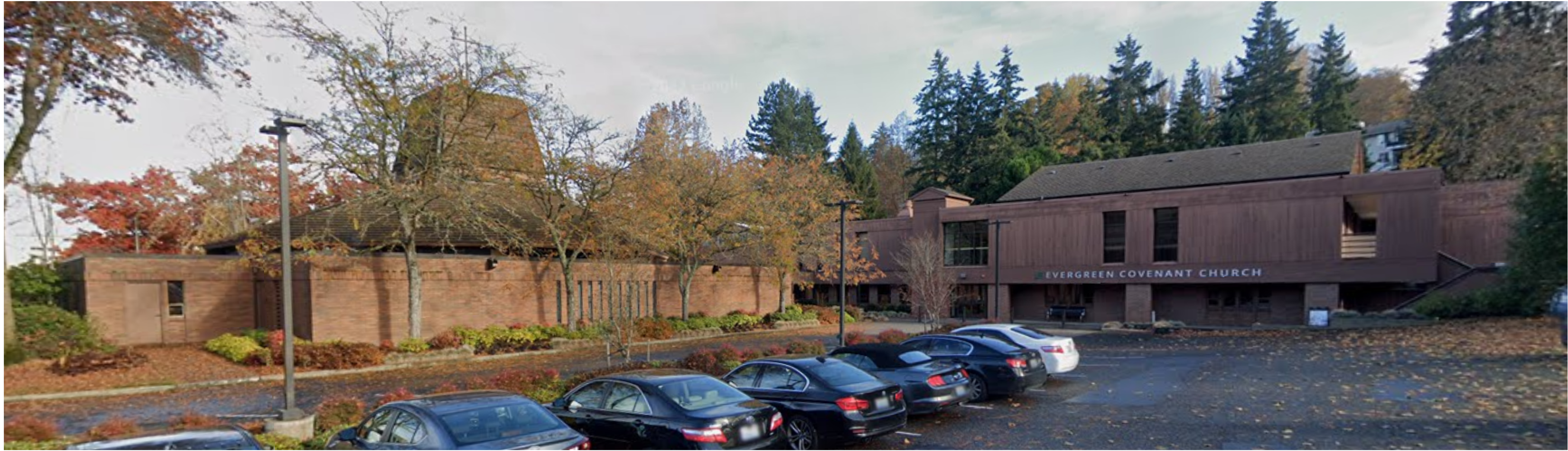
SOUTHERN PARKING LOT VIEW - FACING SOUTHERN PART OF SANCTUARY AND ENTRANCE TO CHILDREN'S WING
